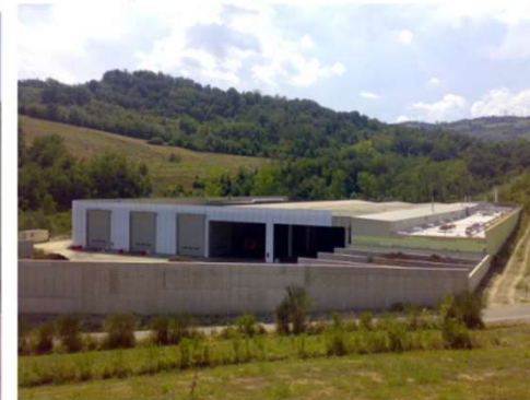
Centralized industrial plants
